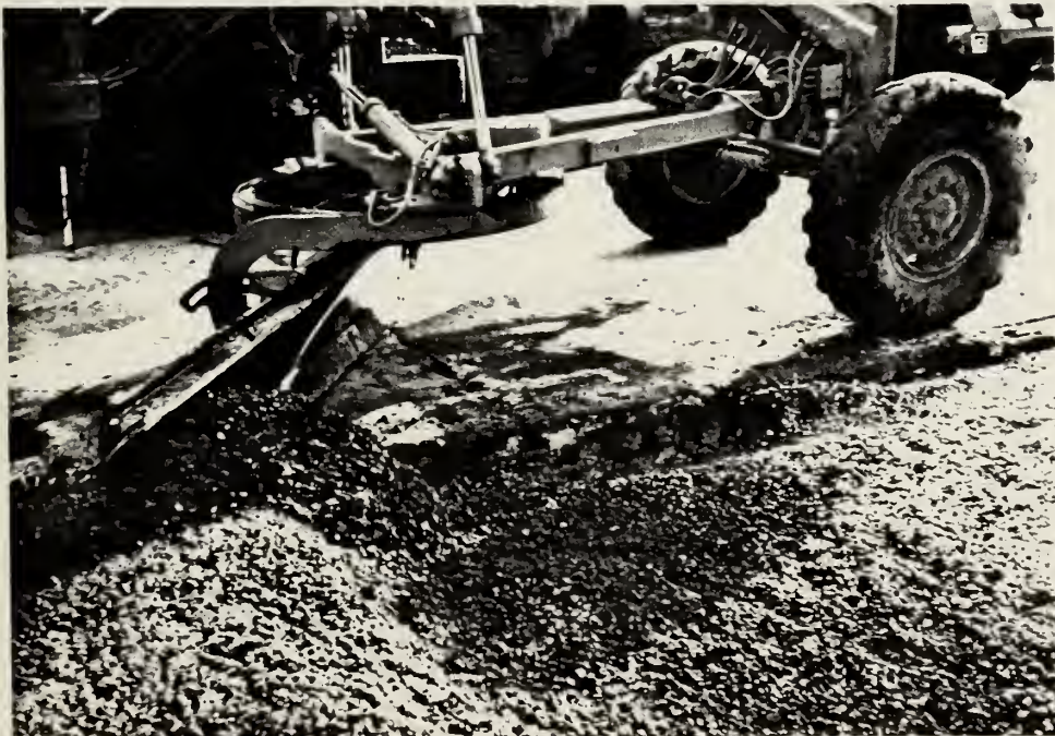
Figure 2.20 Grader Windrowing Wet Mixed Material
